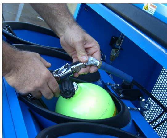
Step 17: Remove fill whip from cylinder.
