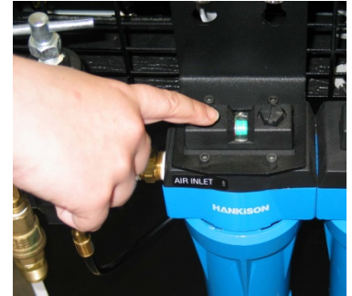
DP Indicator Changes from Green to Red as Filter Ages. Do Not Use When Red.
