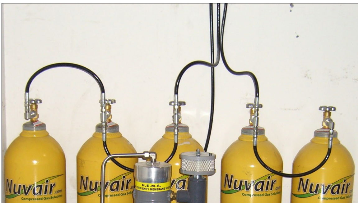
Figure 6. Typical multibank system.
